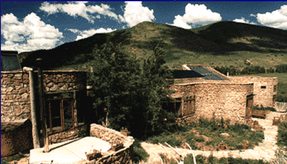
RMI's HQ—a 99%-passive-solar banana farm at 7100'
