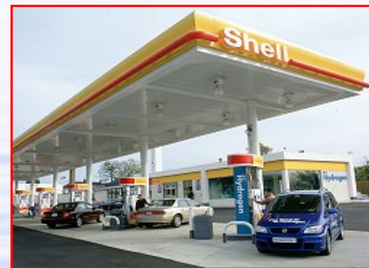
Washington, DC Hydrogen Fueling Station
