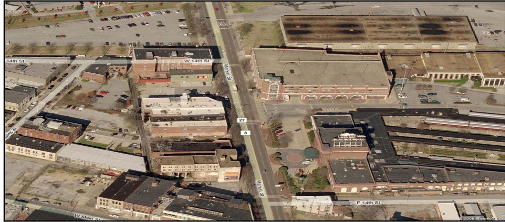
Figure 14. CARTA Electric Bus Facility
