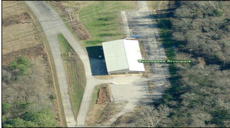
Figure 12. CETE Advanced Vehicle Test Facility Building
