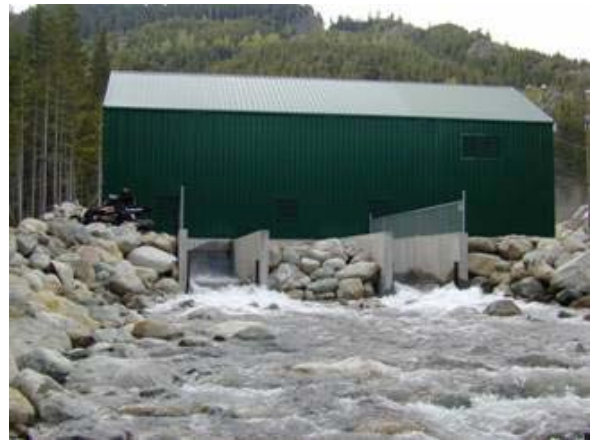
Powerhouse Brandywine Creek
