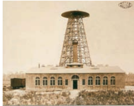
Fig. 2 – Tesla's Wardencllyffe Tower located in Shoreham, Long Island, New York, USA
