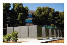
California's Bloom Energy has enjoyed significant interest in its SOFC systems for large stationary applications in the last year. Technological improvements in the hotbox have seen the company's standard offering increase from 100 kW to 200 kW and the addition of a Delaware manufacturing facility in 2012 will open a customer base on the US East Coast.
