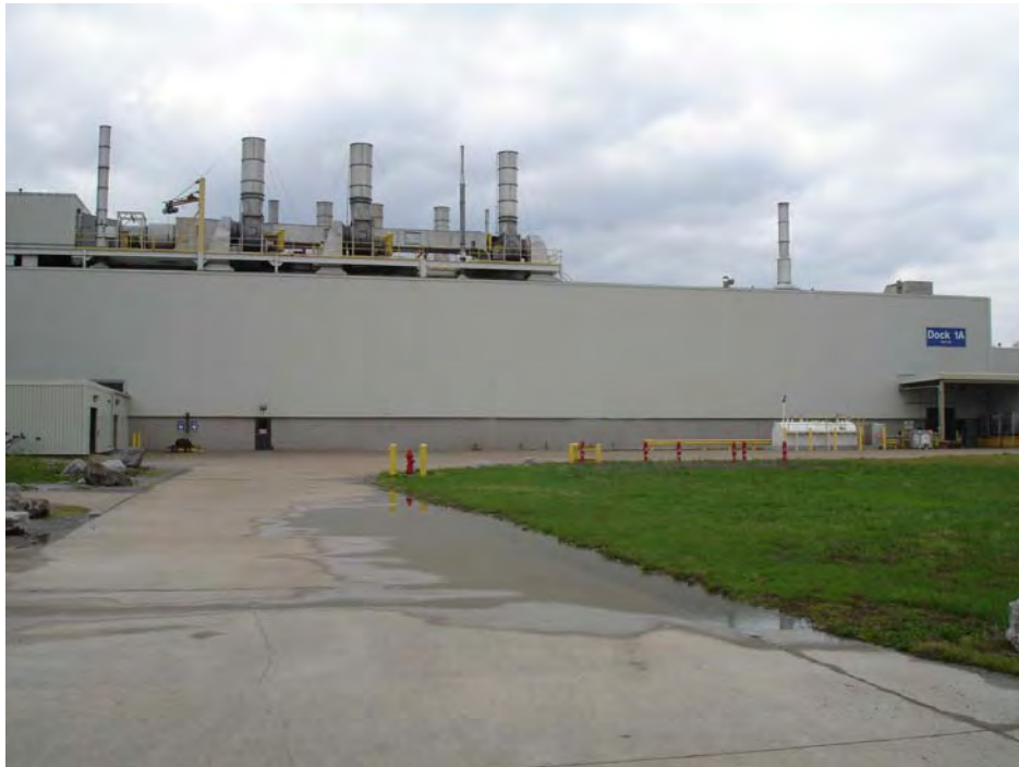
Site for the Potential Fascia Plant Expansion
