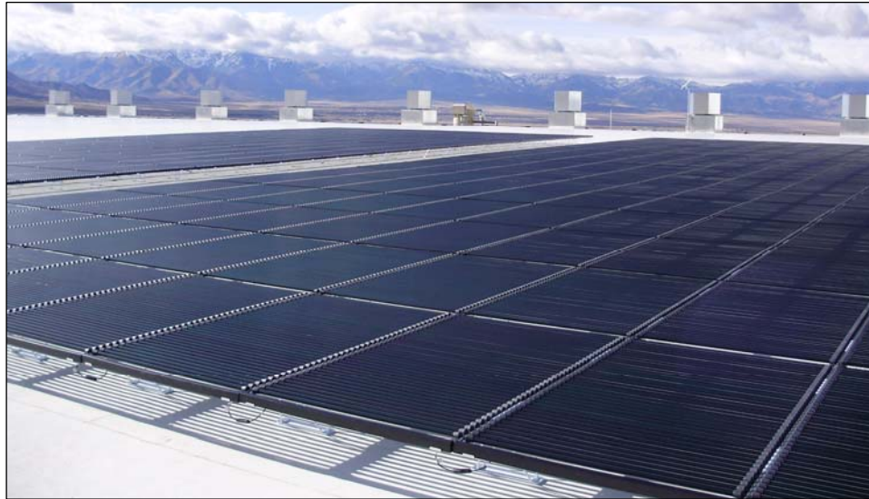
Figure 2-2 Solyndra Rooftop Installation
